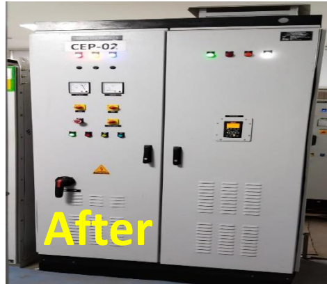
110 KW CEP VFD drive - installed for CEP pump
