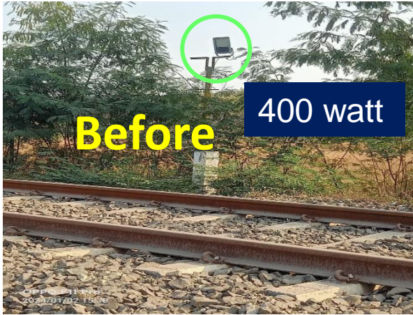
200 W LED fitting in place of 400 W Sodium vapor fitting ( 48 no's )
