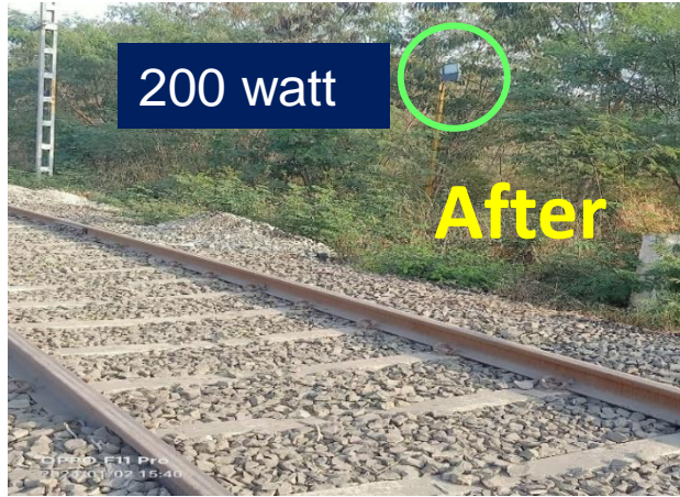
200 W LED fitting in place of 400 W Sodium vapor fitting ( 48 no's )
