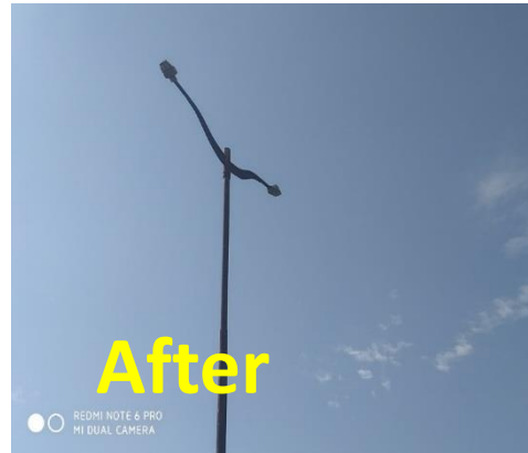
70 W LED fitting in place of 250 W Sodium vapor fitting ( 65 no's )
