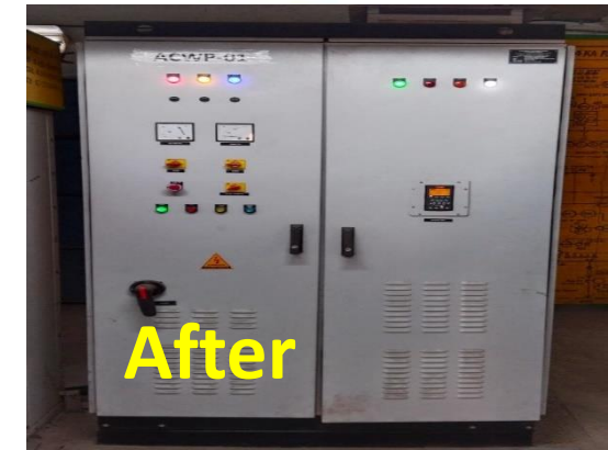
110 KW ACW VFD drive - installed for ACW pump
