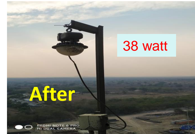
38 W LED fitting in place of 70 W Sodium vapor fitting ( 140 no's )
