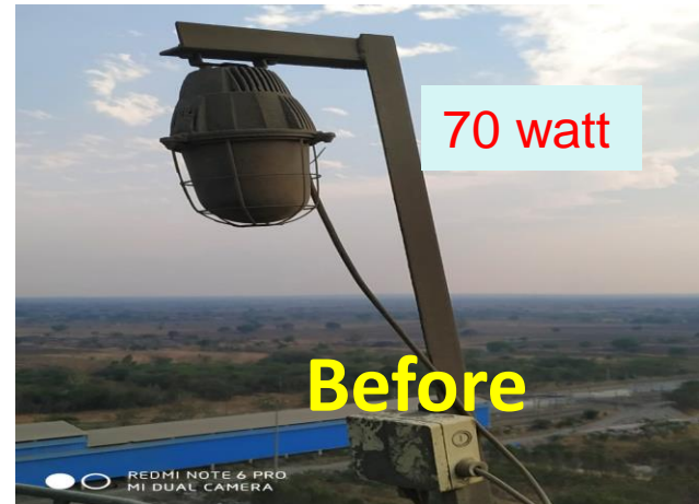
38 W LED fitting in place of 70 W Sodium vapor fitting ( 140 no's )
