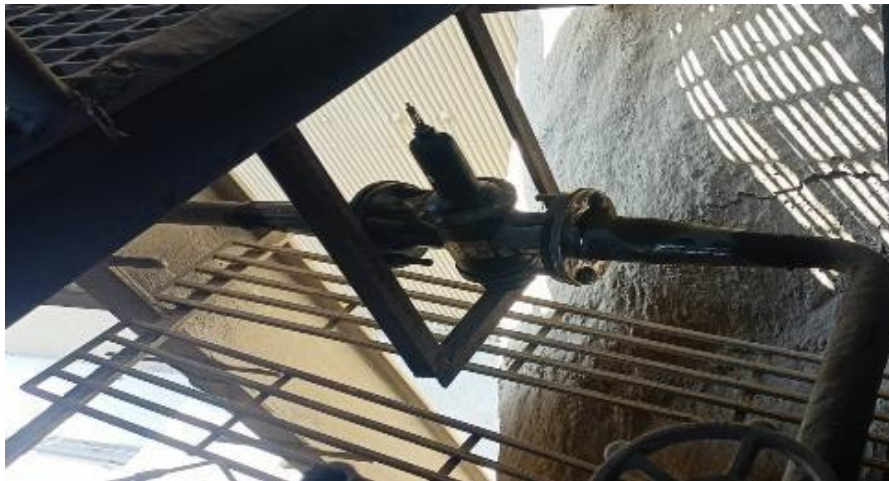
Installation of Pressure Regulation in Cement mill Bag house header line
