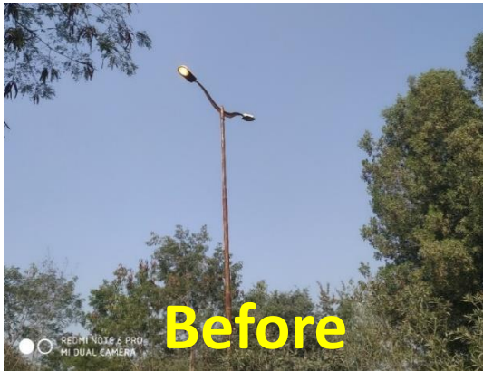
70 W LED fitting in place of 250 W Sodium vapor fitting ( 65 no's )
